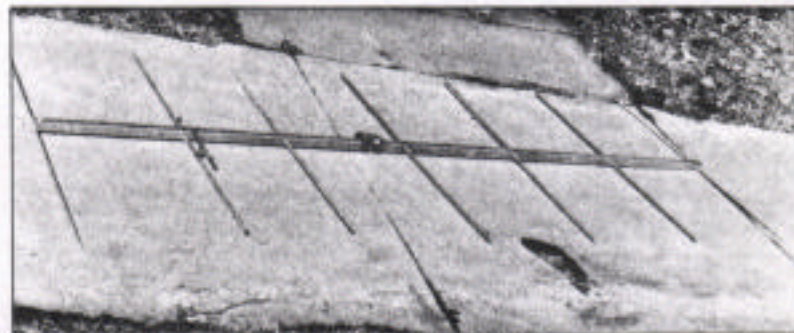
Photo E. The completed beam.
