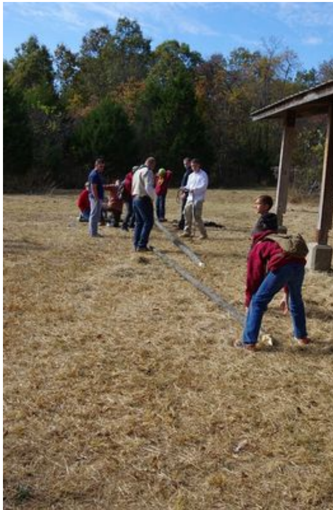
Building the antenna mast
