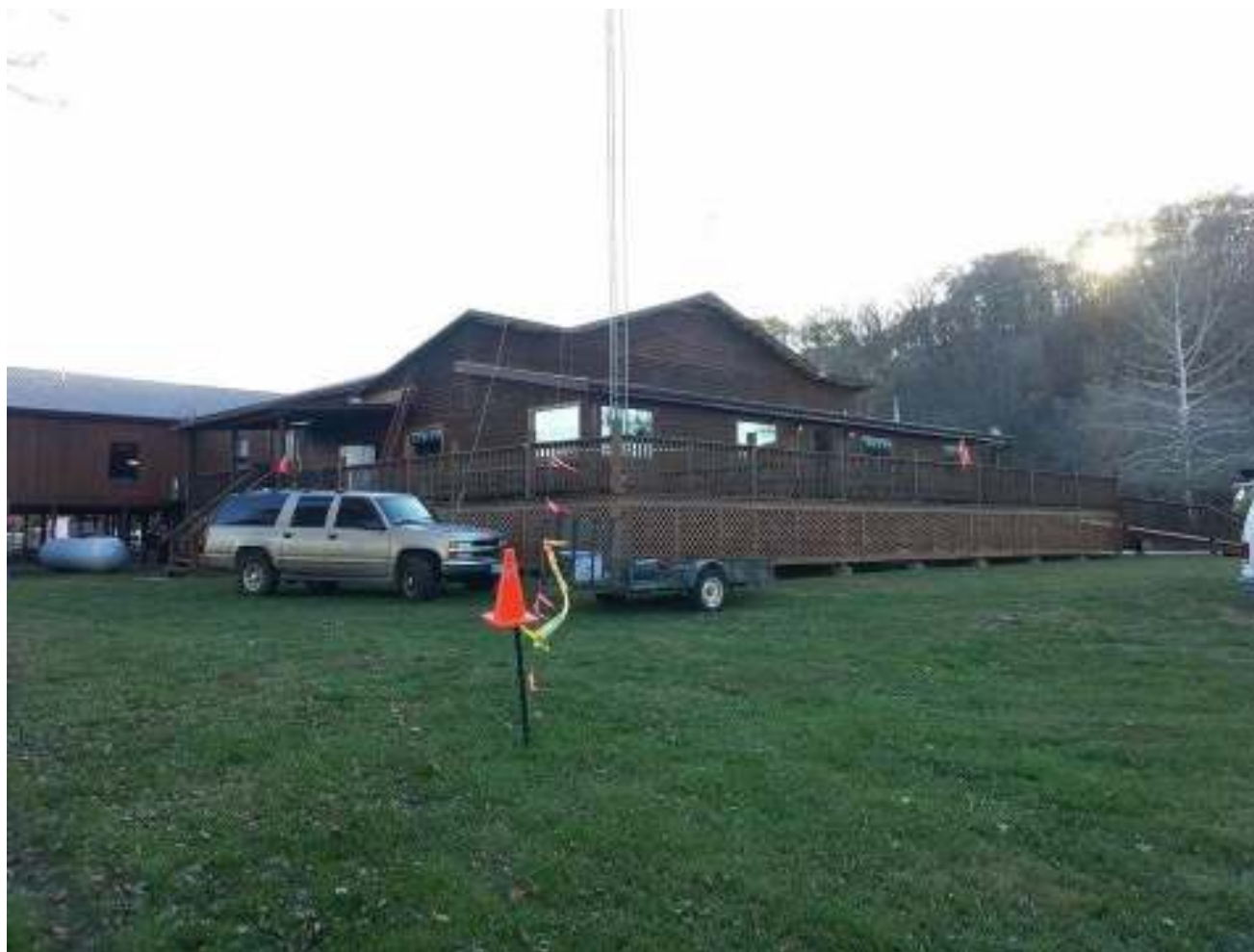
Net control mast and guy wire installation at HQ
