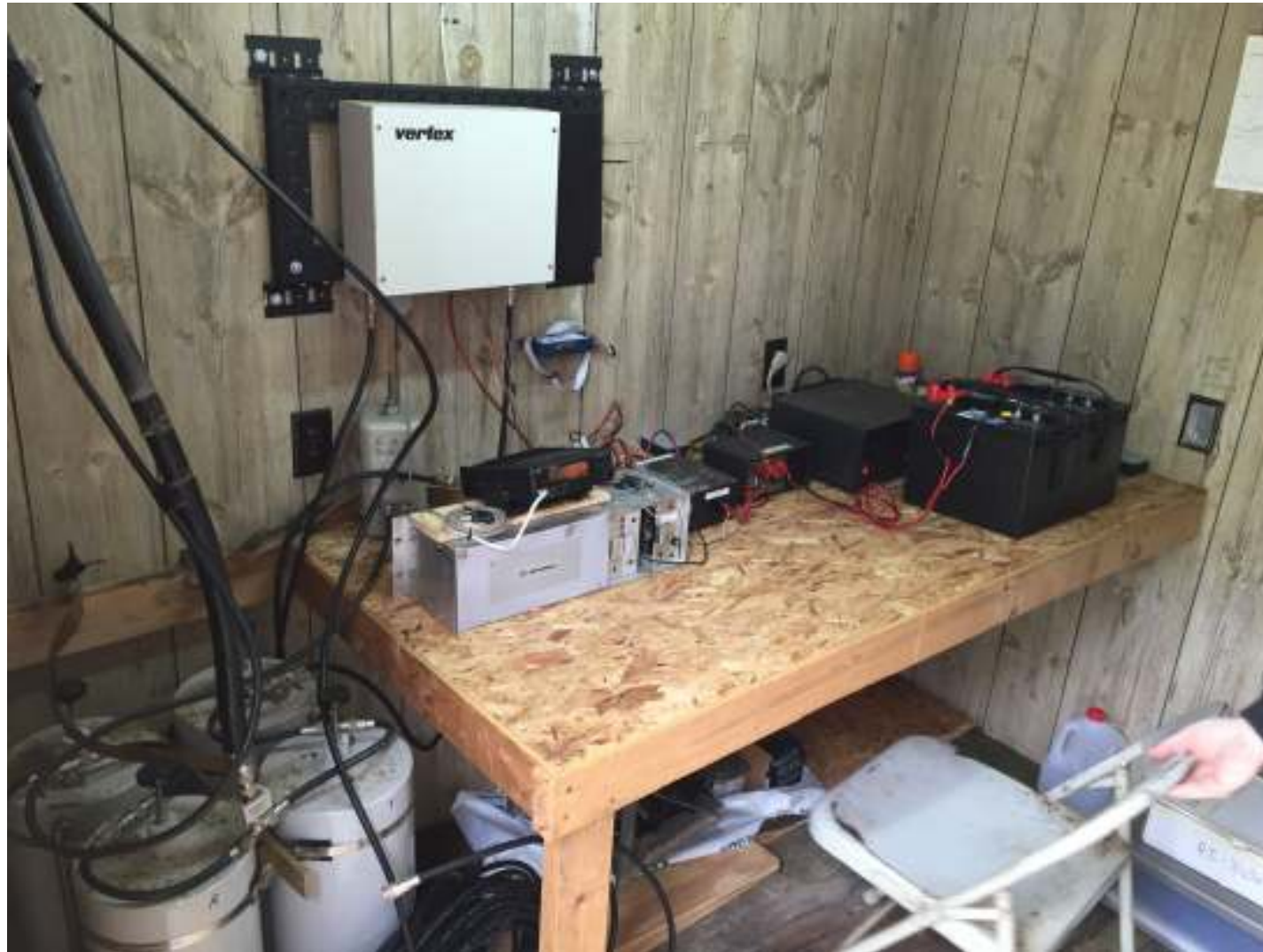
Hancock Repeater: Top Secret Control Room
