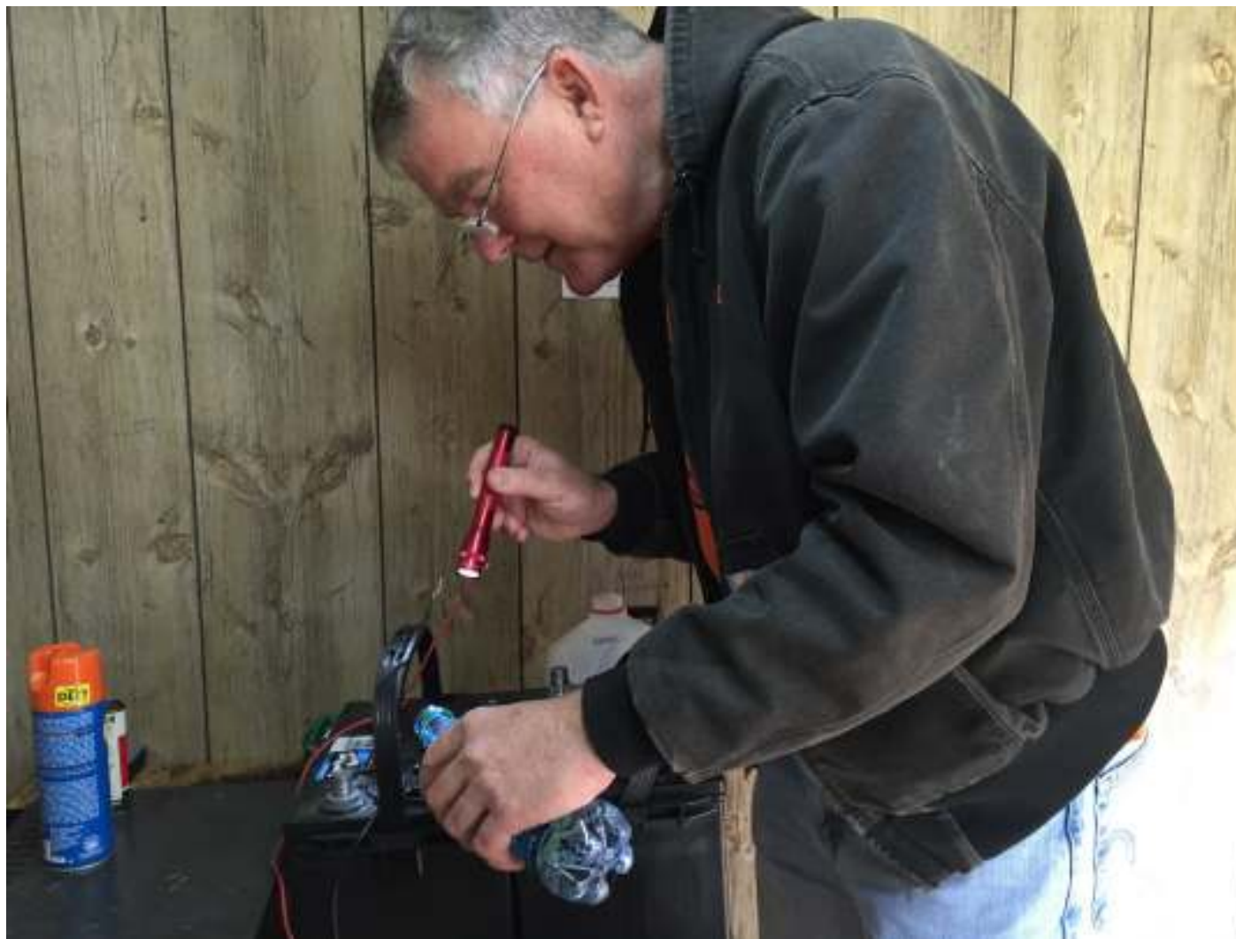
Battery Maintenance: Steve N6RHQ adding DI water to cells
